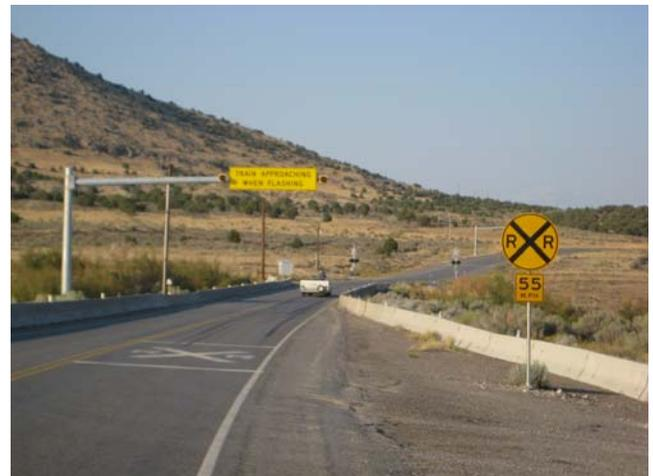
adequate notice to motorists when a train is approaching the crossing. The sign is a black on yellow rectangular warning sign with the legend, "Train Approaching When Flashing." The sign is strategically located to provide
